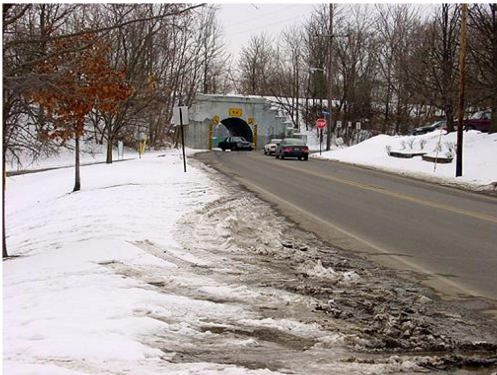
Henry Street Tunnel ca. 2003
