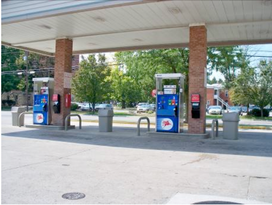
Smell of gasoline and garbage ☹️
